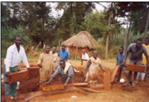
Making bricks for the new church
